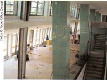
Fotos © Tecno Office Consult
