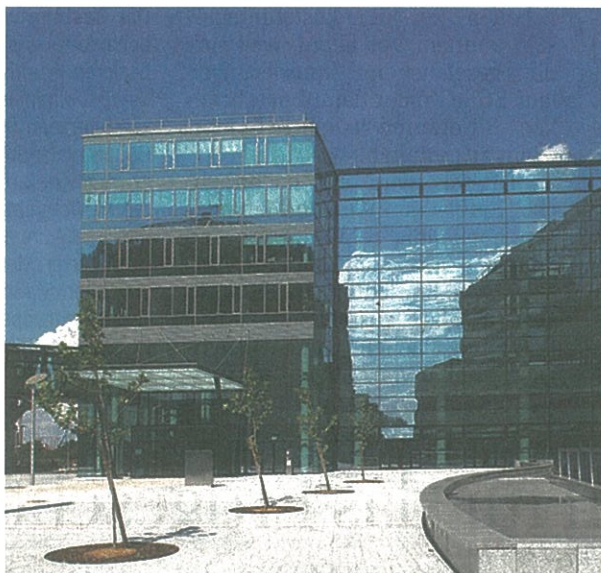
OFFICE CAMPUS GASOMETER
